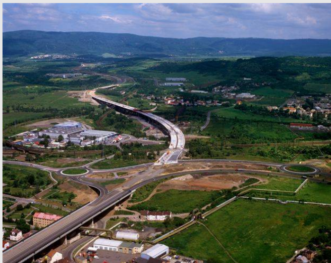
Picture No. 12: Part 0807 of D 8 starts by Trmice bridge constructed on original dumping hoppers coming from opencast collieries A typical town crossing connecting D 8 to four lanes roadway to Usti nad Labem
