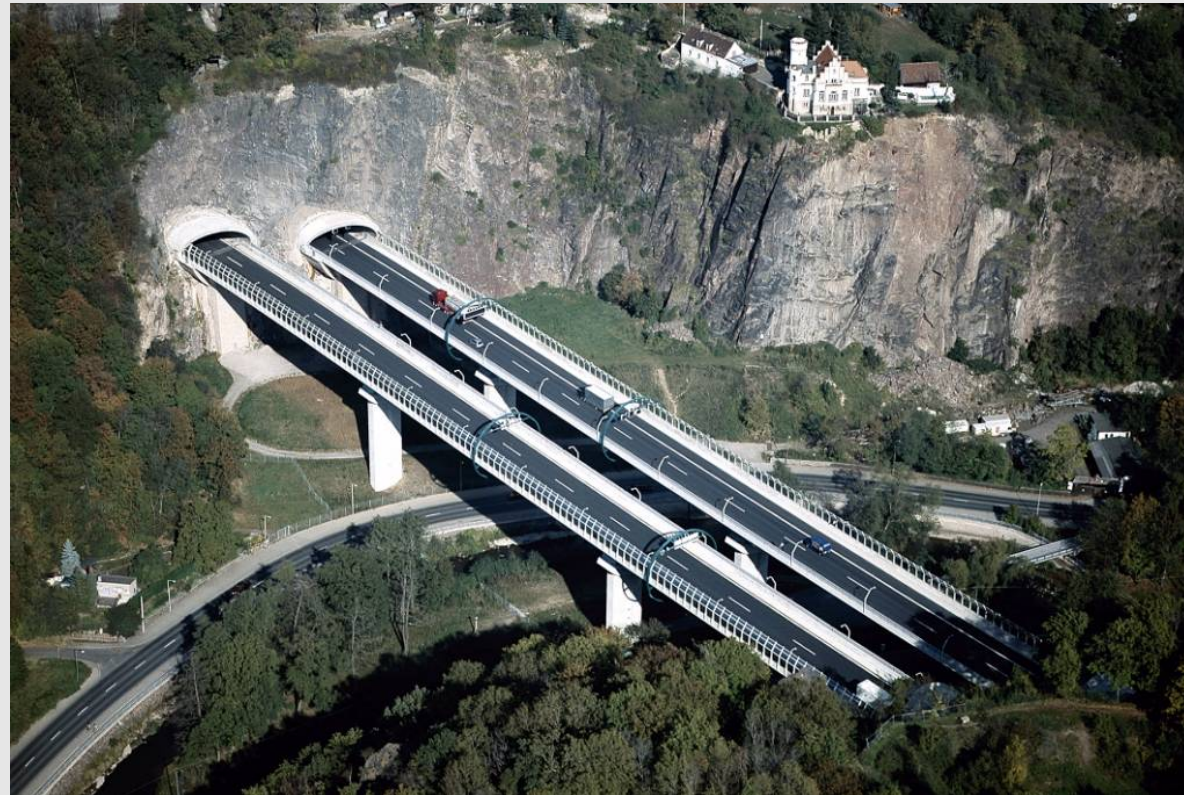
Picture No. 14: South portal of Tunnel Dölzchen and connecting Bridge over Weißeritz-Valley (A 17) Girder bridge, two superstructures, steel-concrete bridge, length 218 m, height 35 m
